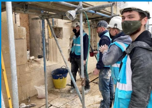
Masons working on the north elevation of the North West Tower
